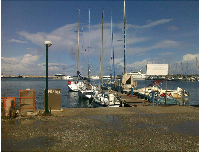
View of pier G – Marina of Rethymno
